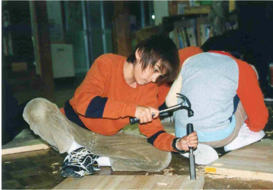
Akira working on the building of the café
